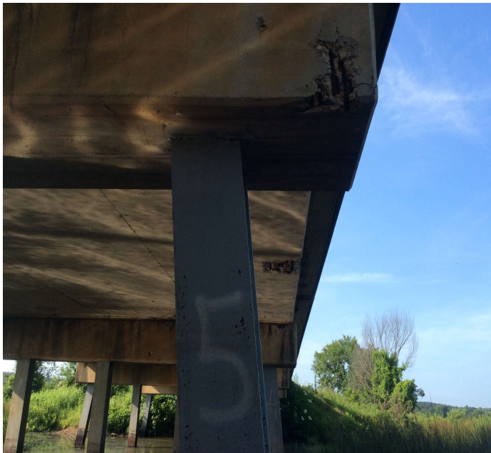
PHOTO 1 Description Bent # 5 Lt spalling with exposed reinforcing steel on the bottom of the cap.
