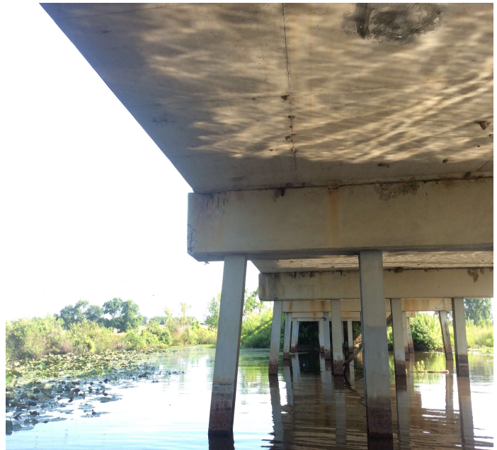
PHOTO 2 Description Bent # 14 Lt cap spalling with exposed reinforcing steel. 12
