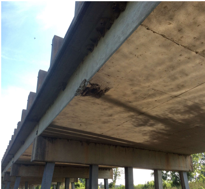
PHOTO 1 Description Span # 4 Lt spalling with exposed reinforcing steel.
