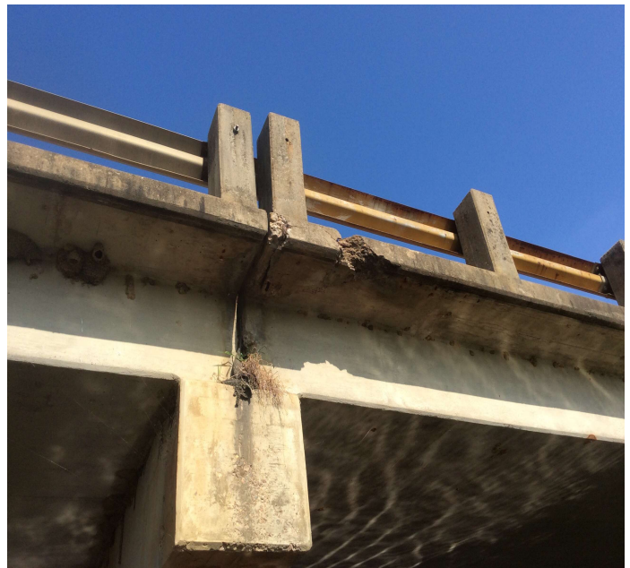
PHOTO 2 Description Span # 17 RT fractured rail post.
