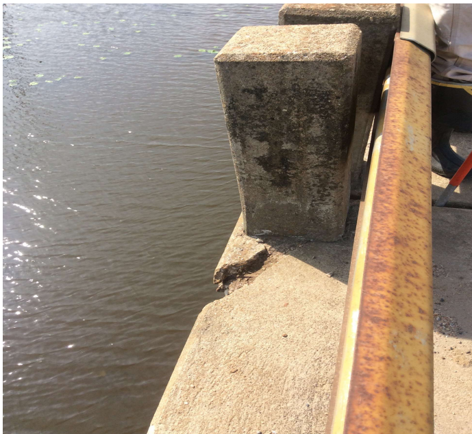
PHOTO 1 Description Fractured bridge rail post located over span 17 right
