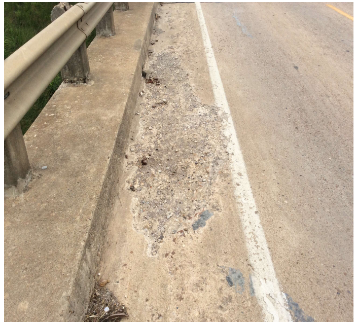
PHOTO 2 Description Span # 5 Lt gutter concrete deterioration.
