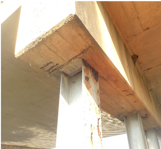
PHOTO 1 Description Bent # 5 Column # 5 active corrosion with section loss.
