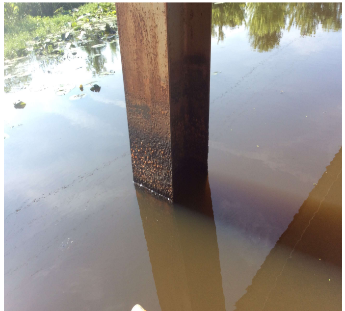
PHOTO 2 Description Heavy pitting at the column bases.
