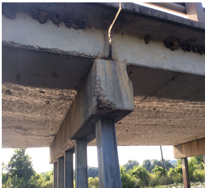
PHOTO 3 Description Bent # 17 Lt end of the cap spalling with exposed reinforcing steel.
